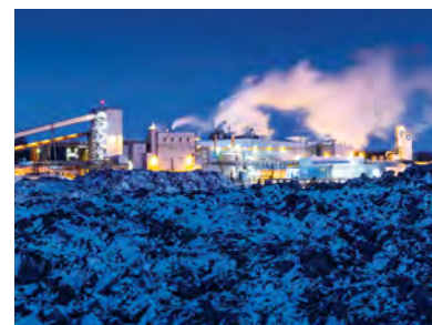
Since 2014, the Kittila Mine has been successfully recycling the waste heat it recovers from its plants and processes to help reduce the mine's overall energy needs and costs.
