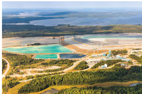
Tailings storage facilities at the LaRonde Complex.
