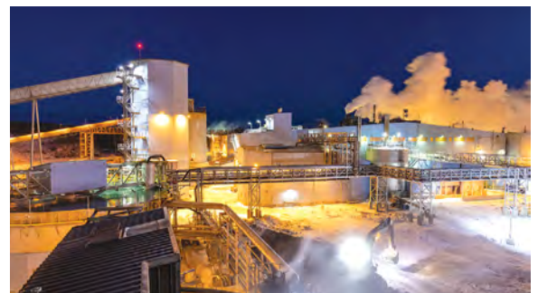
Kittila mine’s heat recovery helps reduce its energy needs and costs.
