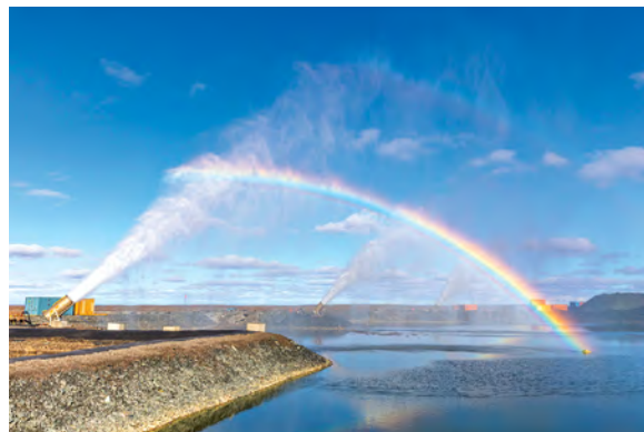
Water evaporators at the Meliadine project in Nunavut are used during the open water season to reduce the volume of saline water stored at surface, thus reducing the potential of saline water migrating within our footprint.
