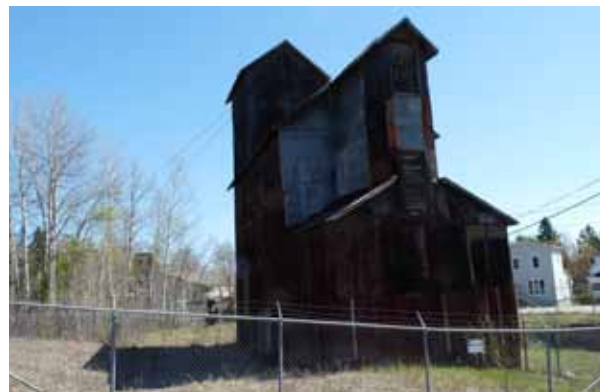
Agnico operated 20 mines in the Cobalt-Coleman area of northeastern Ontario over a period of 33 years. In 2011, we held discussions with various government agencies to determine future remediation work in the area.
