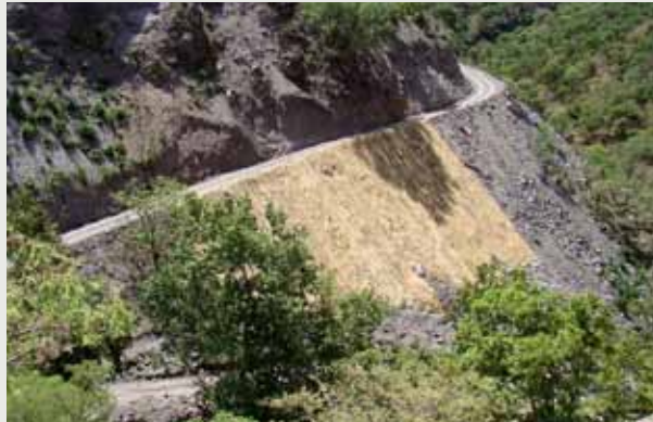
The above picture shows 'malla de coco' partially installed on area.
