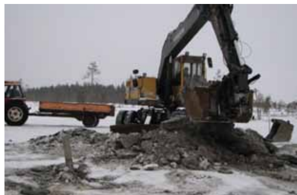
Removing sand and till material after pre-collar drilling.
